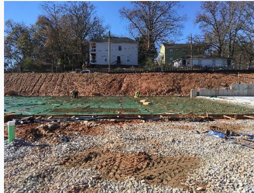
Installing Poly & Wire Mesh at Pour 2
